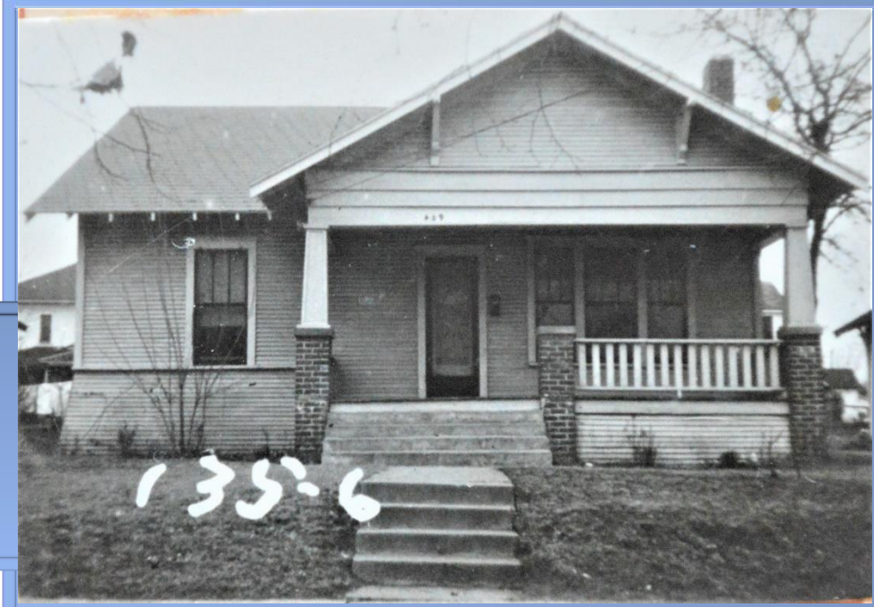
409 Amarillo – McClendon House Craftsman – Built 1919 High Level of Original Integrity
